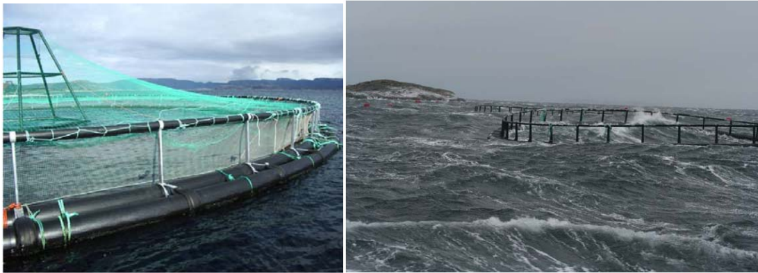
Figure 1. To the left: Details of circular HDPE cages (SINTEF Fisheries and Aquaculture). To the right: Circular floating collar of HDPE without attached net cage in bad weather (David Kristiansen).
